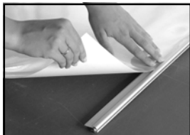
Step C: Firm pressure onto surface
